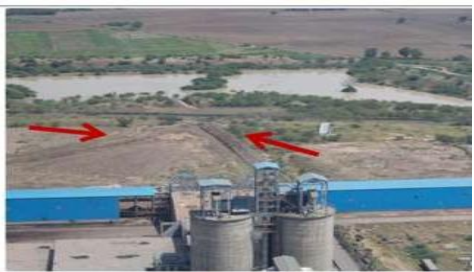
Storm Water Drains connected to Pond
